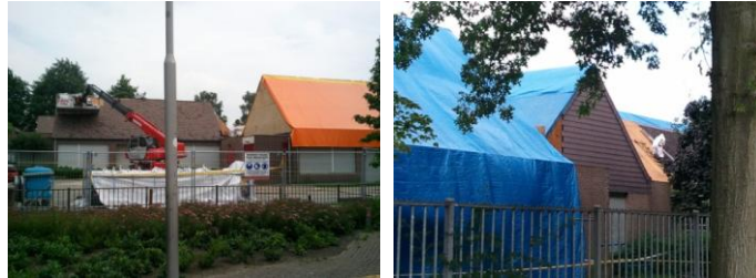
Preventieve asbestsanering school
